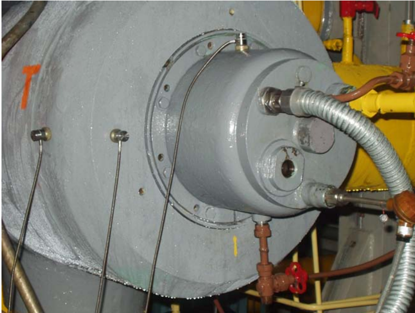
Arrangement piezoelectric sensors on the unit
